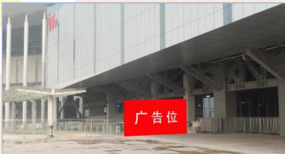
C03 Billboard beside East / West registration hall entrance
